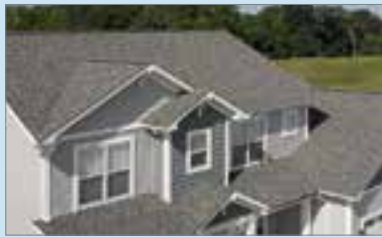
Roofing and Ventilation
