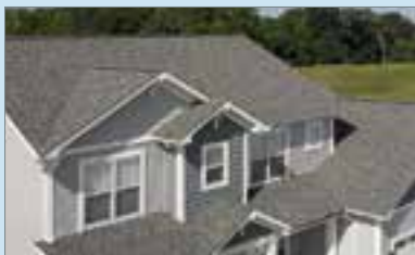
Roofing and Ventilation
