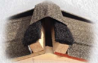
Installed without Center Beam
